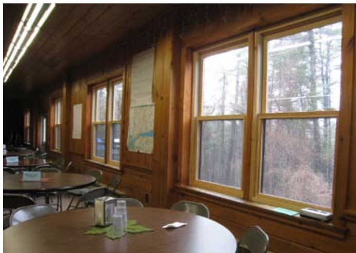
Energy conserving, thermal-paned windows have been installed in the Cedars and Glen.
